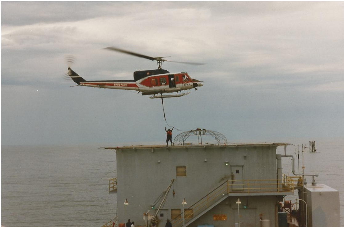
Installing DAS on Platform with helicopter
