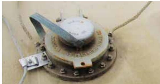
Tinned Copper Flexible Braid Conductors
