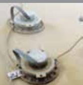
The Streamer Delaying Air Terminal (SDAT), is our most basic type of lightning protection and certainly sufficient for most tank battery installations, however, there are instances that require a higher level of protection and might need a more enhanced product.
