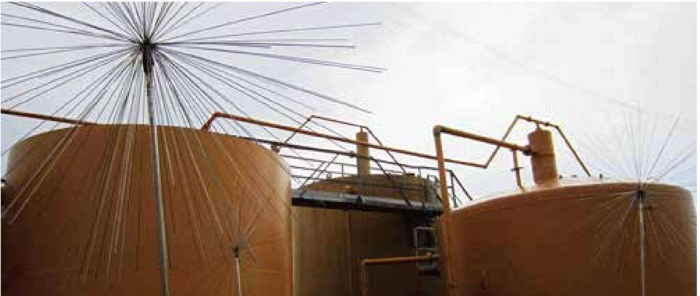
The SBI is a modular lightning prevention component used to supplement Dissipation Array installations, and as the first line of defense for structures that require lightweight protection with a low wind profile.
