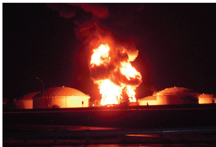
"Tank Explosion at night - Colonial Pipeline Tank Farm Greensboro, NC June, 13, 2010"
