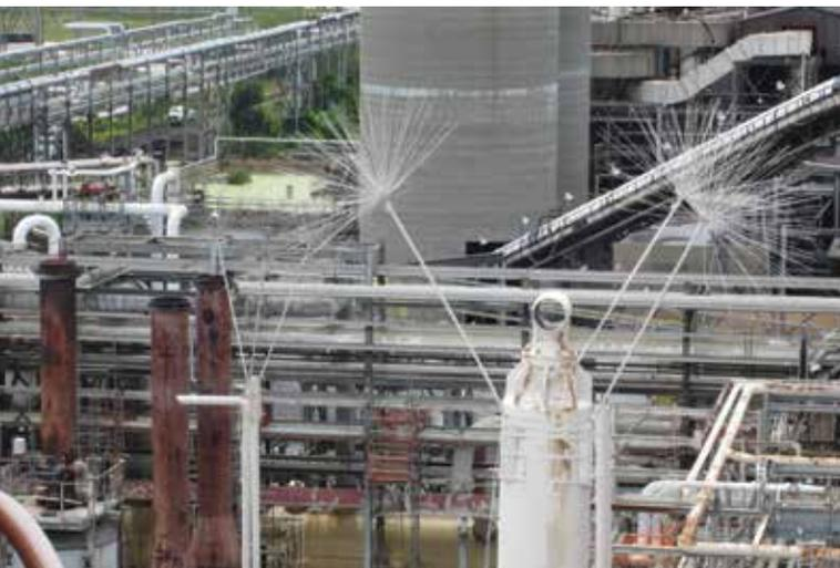
Phillips 66- Spline Ball Ionizers
