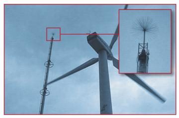
using the storm's energy to develop a dense corona plasma. As the electrical field grows, this highlycharged corona becomes more attractive, drawing strikes safely to the IPG and preventing damage to valuable assets.
