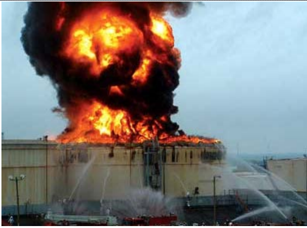
Losses from an oil storage tank explosion caused by lightning can be far reaching. Photo courtesy of Lightning Eliminators & Consultants
