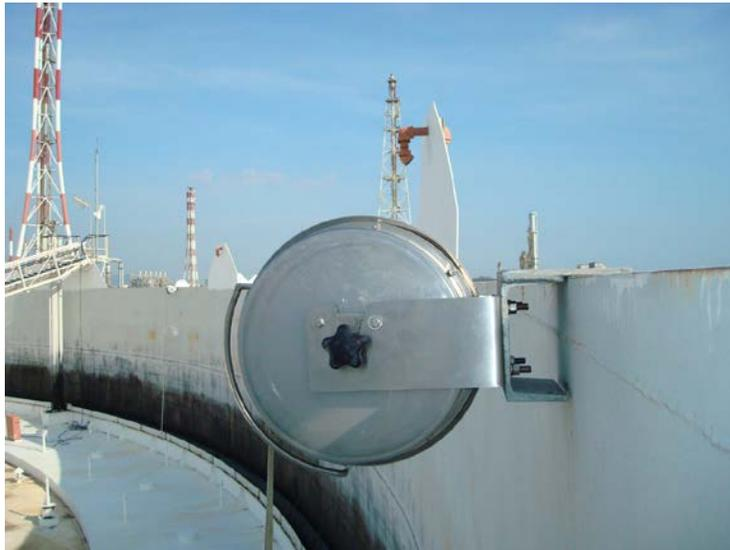
*Lightning Eliminator's Retractable Grounding Assembly RGA®*
