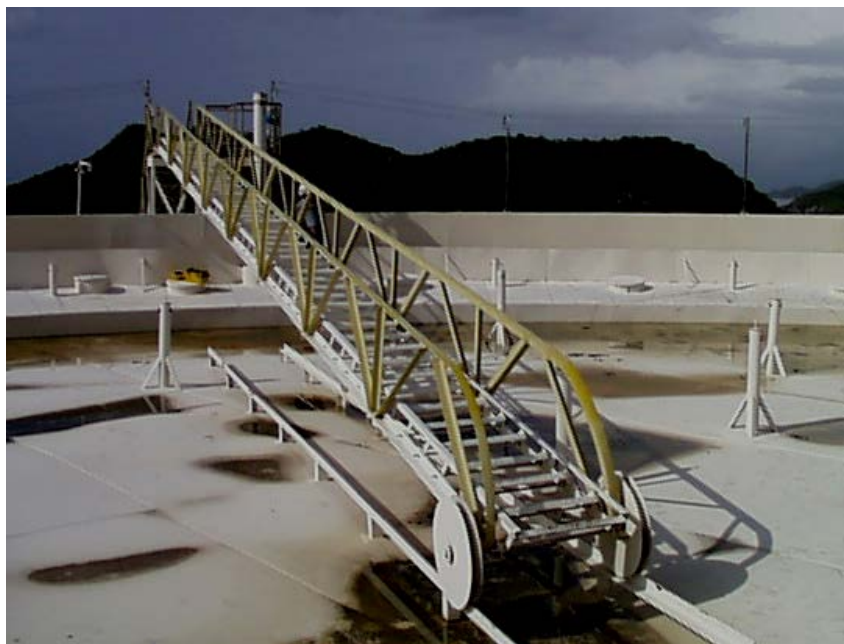
Figure 8: Walkway on FRT
