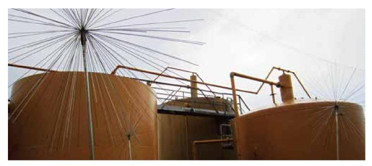
The SBI is a modular lightning prevention component used to supplement Dissipation Array installations, and as the first line of defense for structures that require lightweight protection with a low wind profile.
