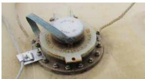
Tinned Copper Flexible Braid Conductors
