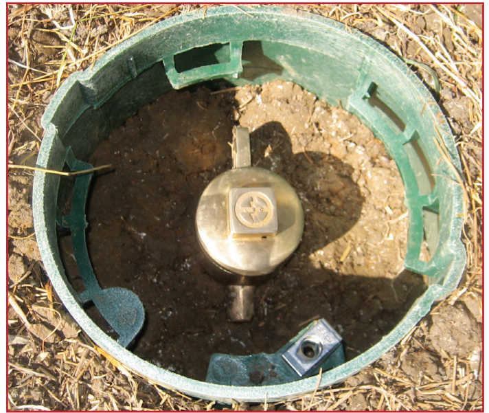
Chem-Rod grounding electrode installed in service well.
