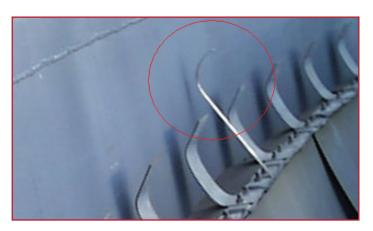
Substantially reducing the risk of sustained arcs requires a reliable, full-time, low-impedance and low-resistance connection between the tank shell and roof. Additionally, the connection must operate regardless of the tank wall's condition.
