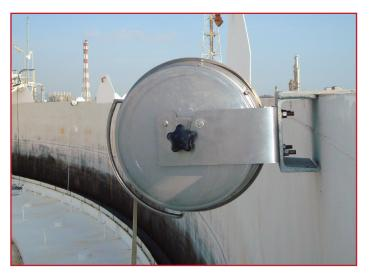
(FRT). FRT's are especially vulnerable to the direct and indirect effects of lightning. A direct or a nearby lightning strike will cause electrical currents to flow across the tank shell and roof. When these lightning currents arc across the roof/shell interface, they can ignite any flammable vapors that may be present. It is therefore necessary to bond the roof and shell to prevent arcing at the roof-shell interface.
