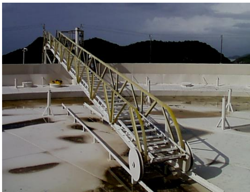
Figure 8: Walkway on FRT
