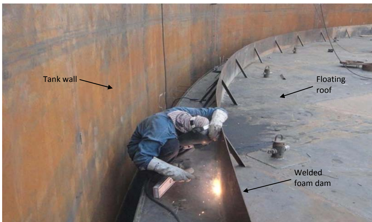
Figure 7: Typical welded foam dam
