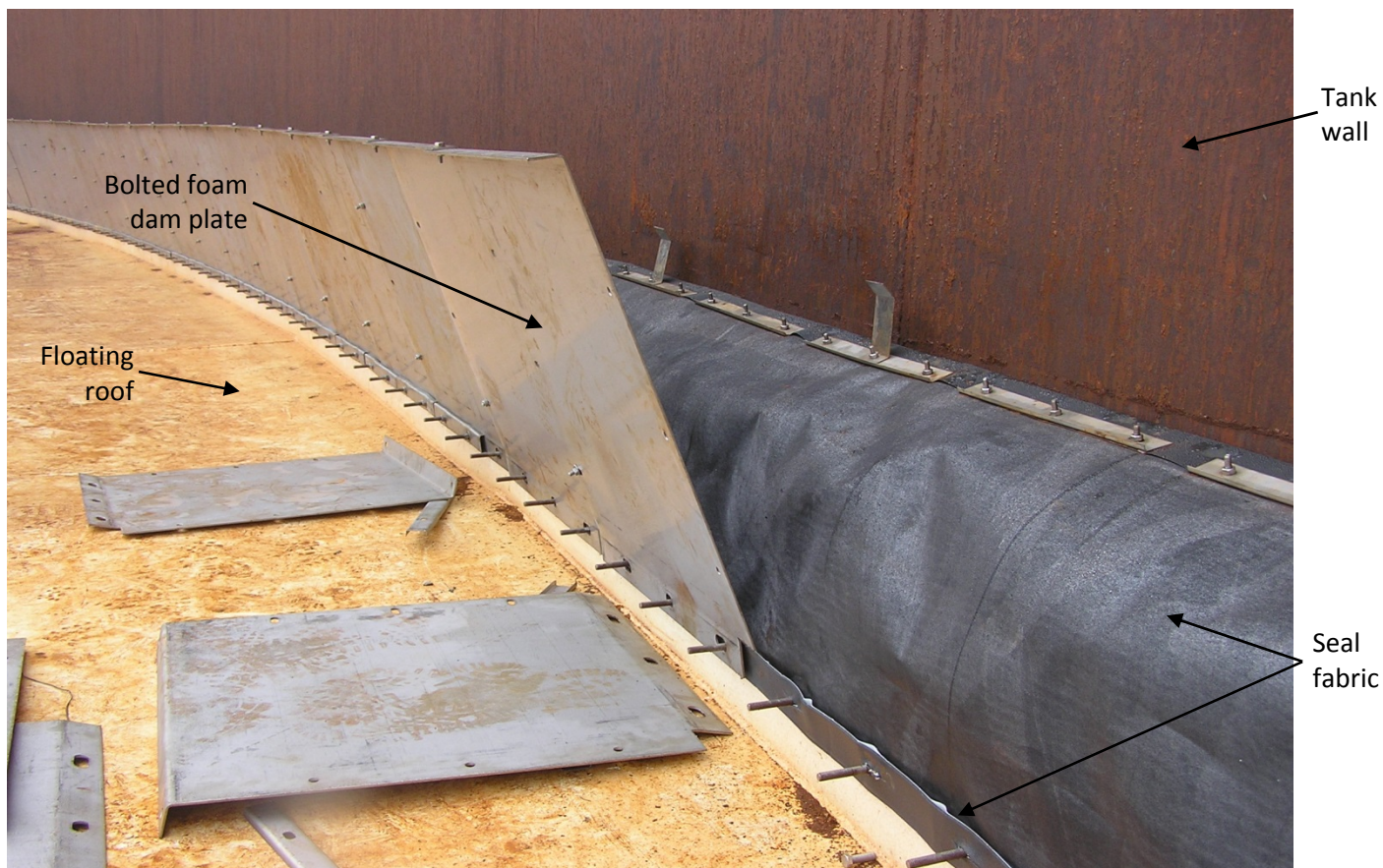
Figure 8: Typical bolted foam dam
