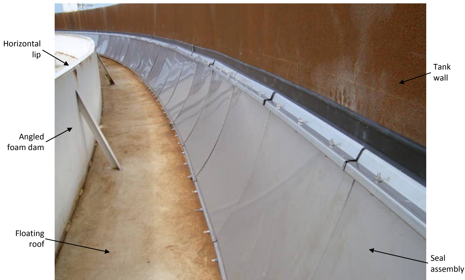
Figure 9: Typical angled foam dam
