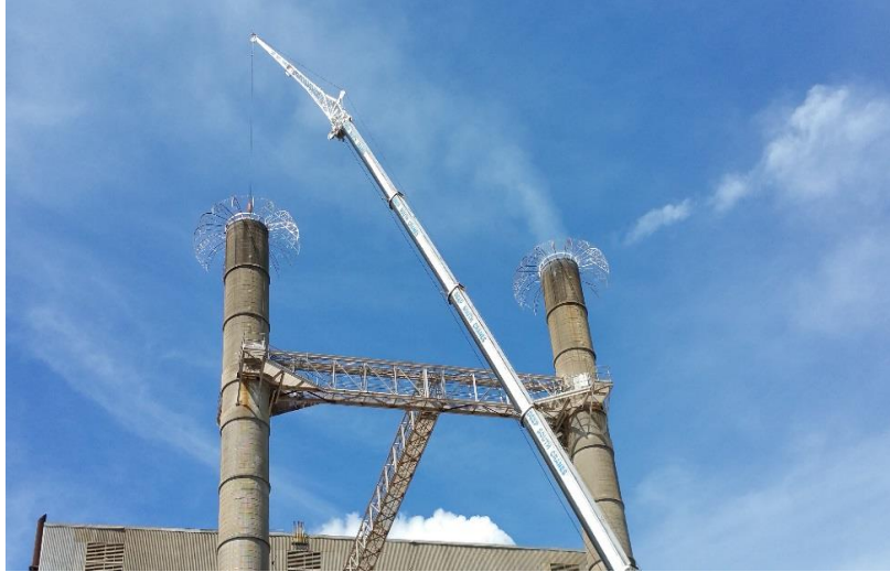
Figure 3: DAS Hemispheres being installed on stacks
