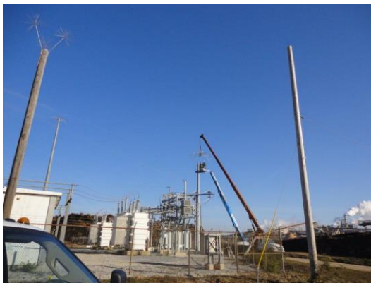
Figure 2: (left) SBI's on pole and DAS being installed on substation; (right) SBT's on switchgear building
