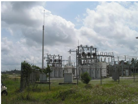
Figure 1: (left) ESE on pole; (right) lightning masts on substation structures
