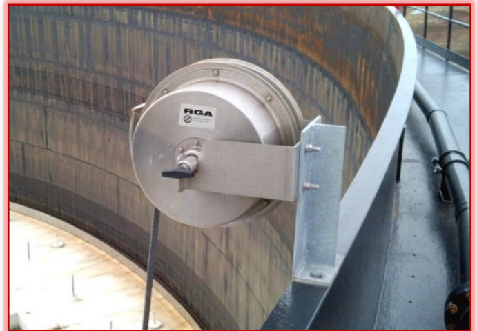
RGAR 750 Generation 2 mounted to a vertical standoff bracket* on a floating roof tank.
